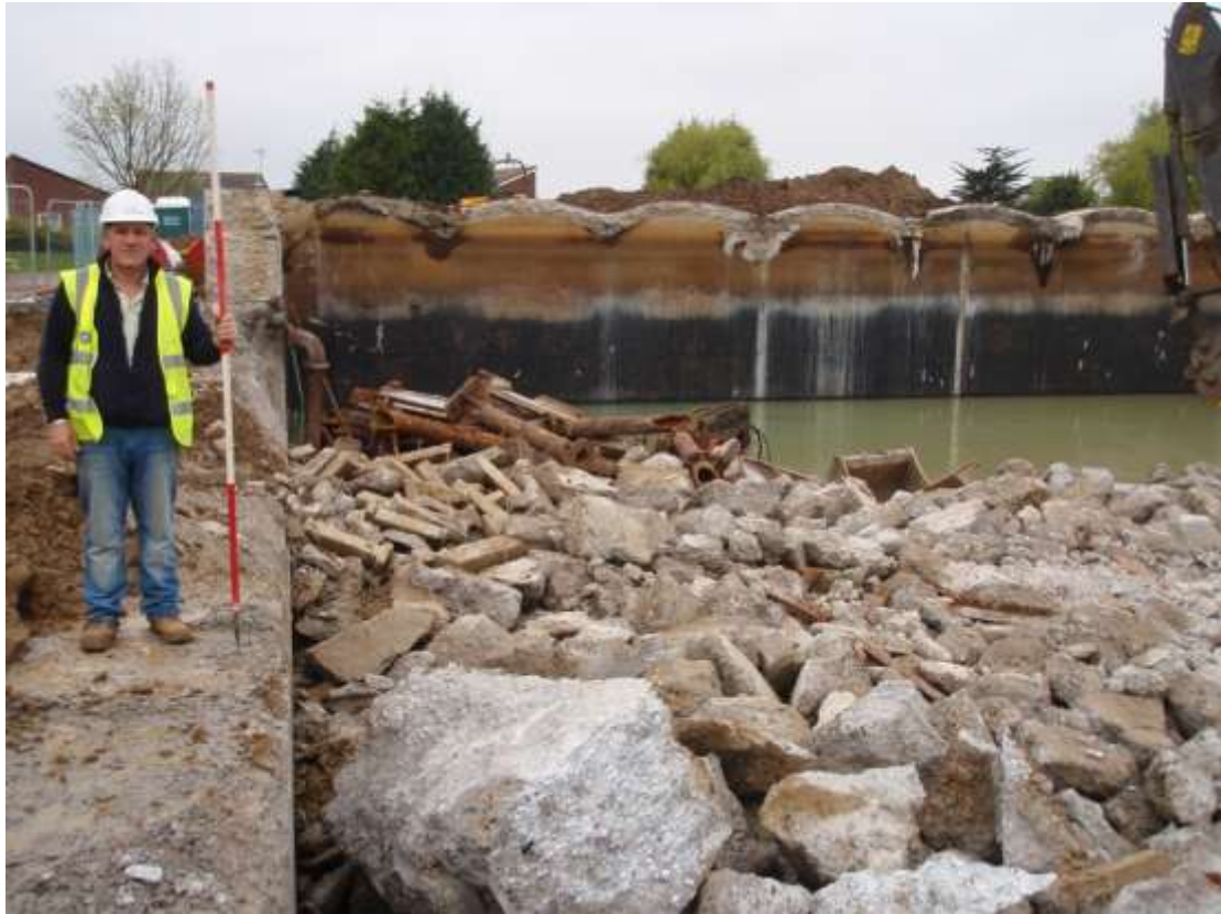
Plate 13. Demolition phase of reservoir (facing west)
